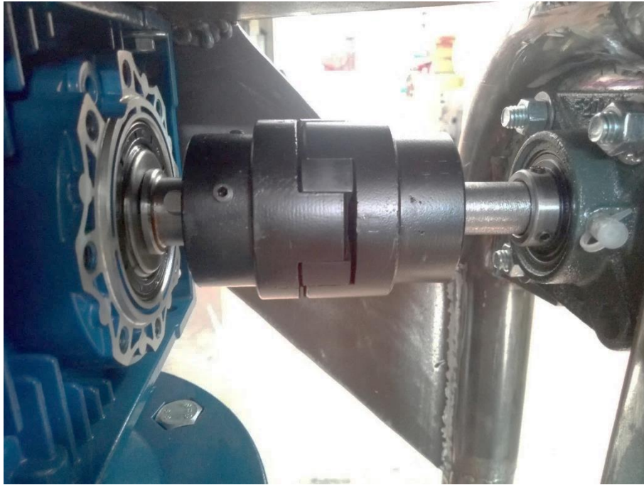
Figura 7.11: Acople flexible Fenner instalado, Vista 1.
